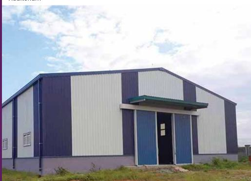
Sahara is a leading designer, manufacturer, supplier and erector of plated portal Pre-engineered Metal Buildings (PEB) in India. We deal in PEBs made of steel that are entirely factory manufactured post designing. Their erection involves the assembling of all the components and the use of bolts on-site, which is extremely time-saving. PEB encompasses all types of constructions, including shop ping malls, factories, showrooms, godowns, auditorium, sports complexes, and even community centers.
